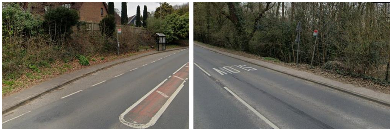
Graphic 5-38 Bus stop facilities on B2177 Winchester Road
