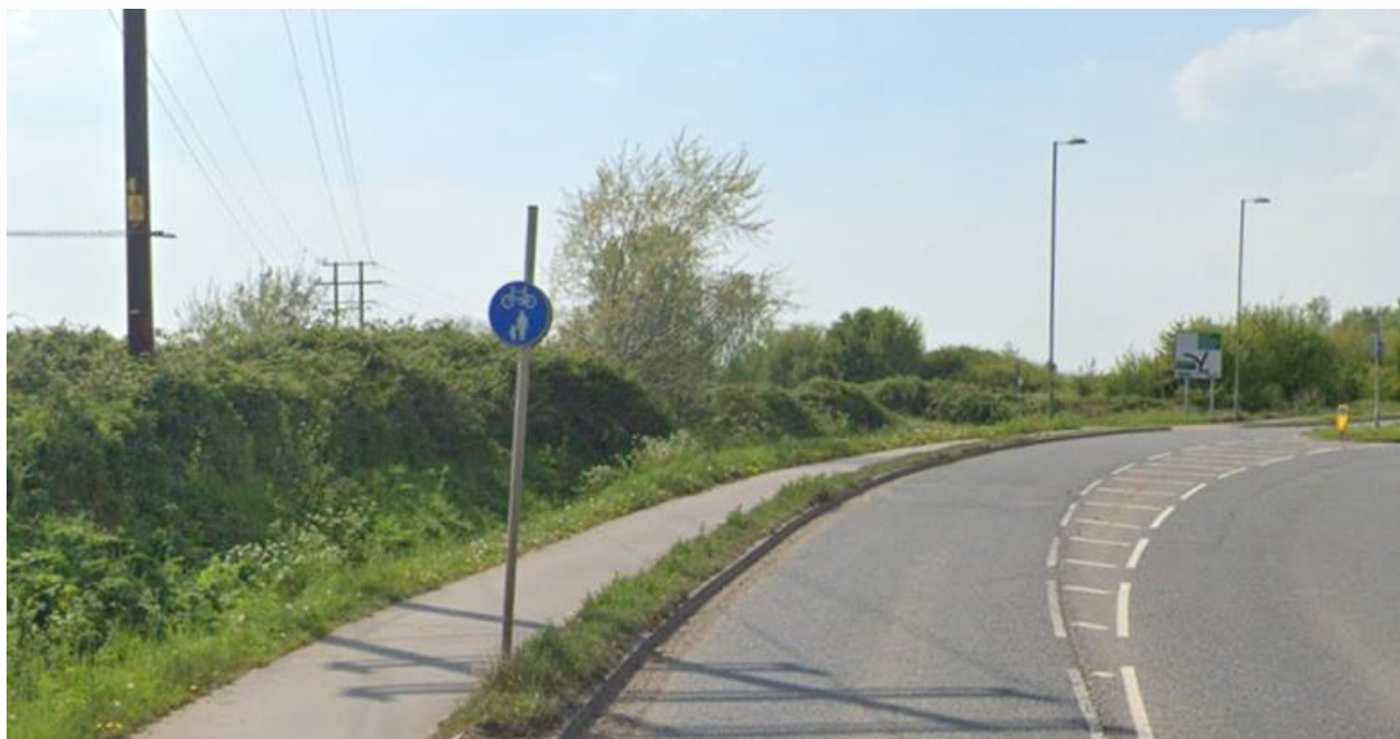
Graphic 5-5 Off-road shared use cycleway on Harts Farm Way
